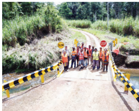
The construction team completes the bridgeworks.
